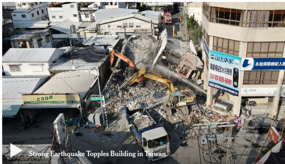
A 6.8 magnitude earthquake in Taiwan killed at least one person and collapsed at least one building in the town of Yuli in Hualien County. Ritchie B Tongo/EPA, via Shutterstock
